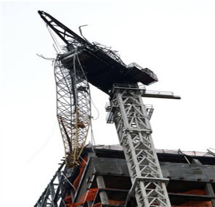
Tower Crane damaged during an extreme storm event and weathervane not actuated.
